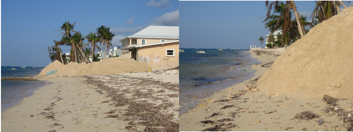
Figures 5 and 6: The DoE responded to a complaint from the public that this stockpiled material was causing considerable turbidity and siltation of the marine environment.
