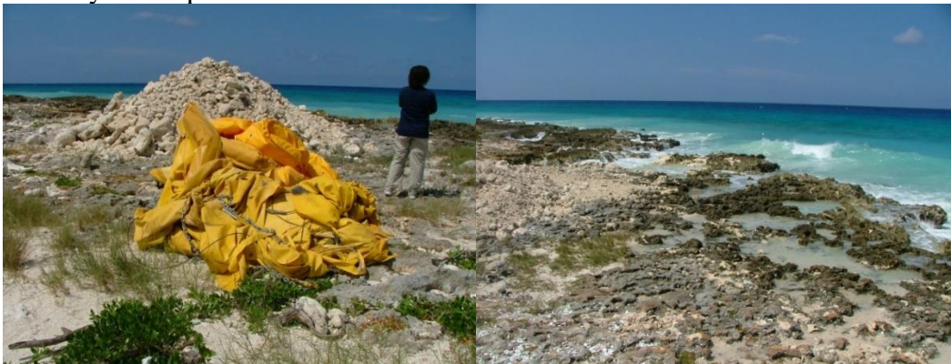
Figures 10 & 11: Material stockpiled on the edge of the water interacting with moderate wave activity and entering the marine environment
