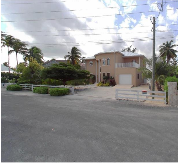
Fig. 1-254 Sand Point Road – Existing property and wood fence.
