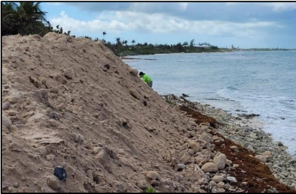
Figure 21: Material stockpiled too close to the water's edge which would or would be likely to enter the marine environment during a storm.
