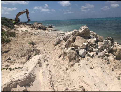
Figure 17: Stockpiling and on-land activities impacting the marine environment through turbidity and deposition of waste
