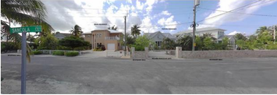
Fig. 6. Street view of 254 Sand Point Road and adjacent property boundary wall and gates.
