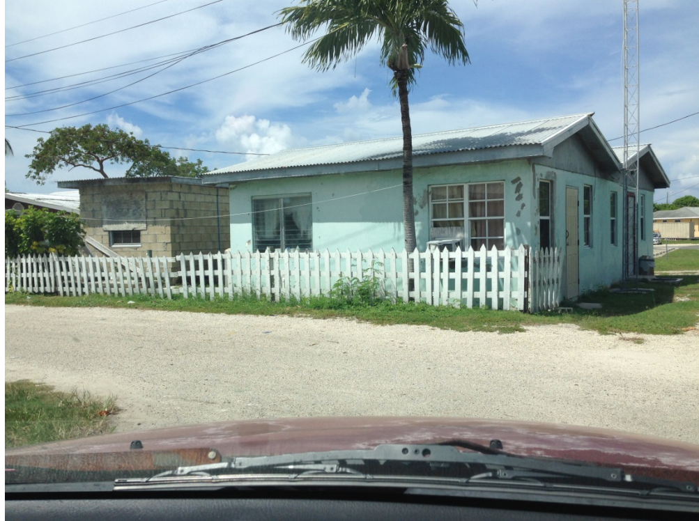
South view of property along Tulip Lane
