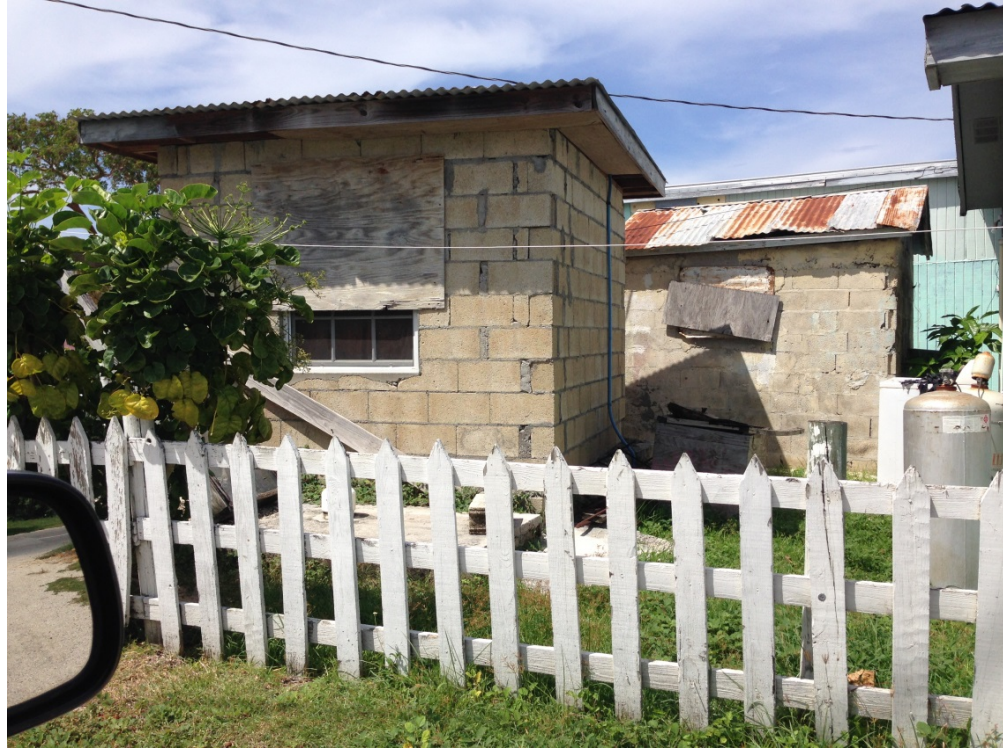
Two unfinished ancillary buildings behind house/duplex
