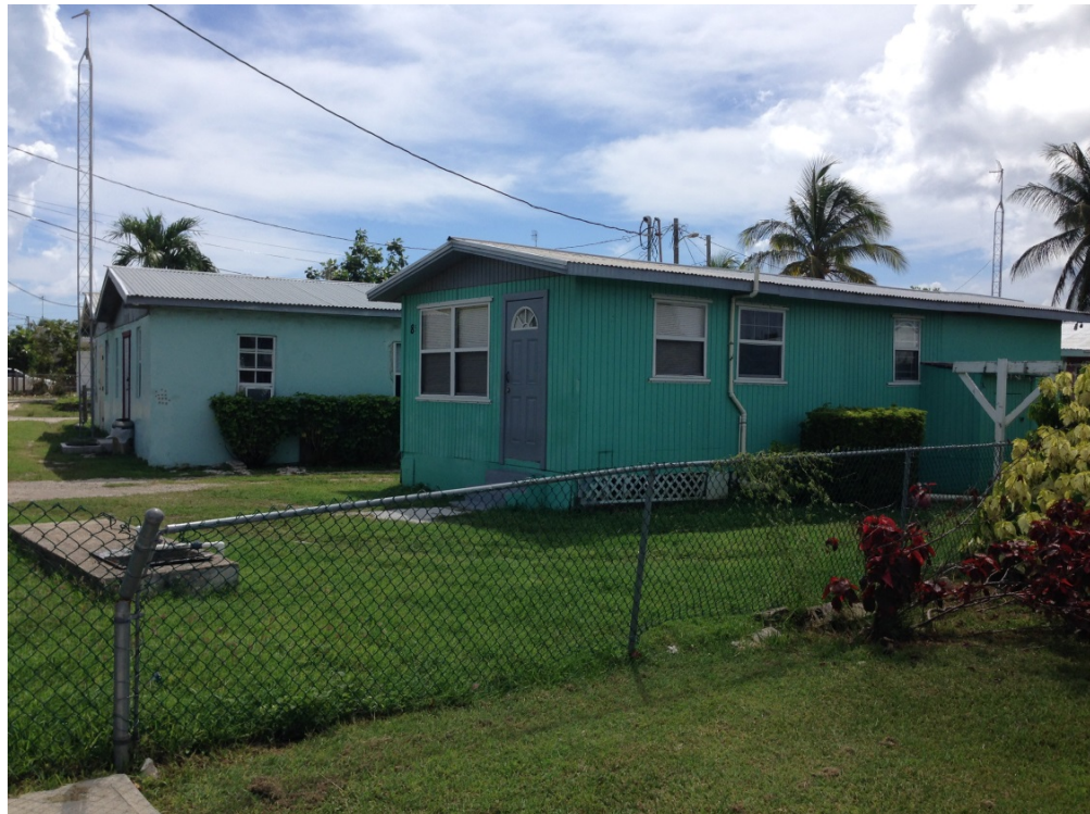
North view of property
