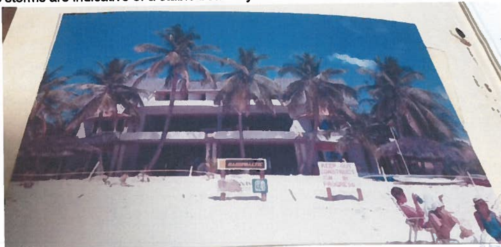
FIGURE 7 –EXISTING WOOD FRAMED CABANAS
