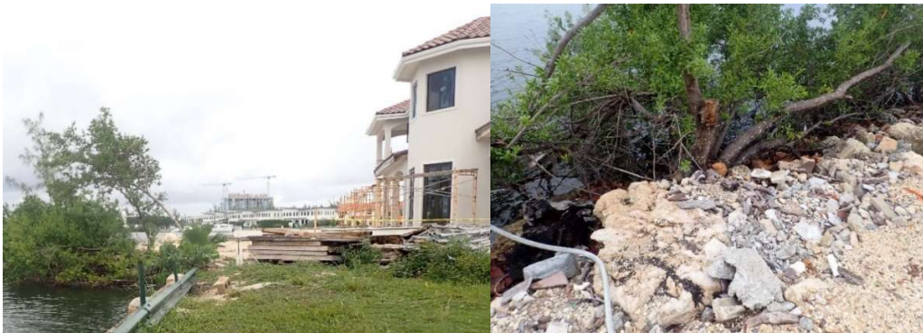
Figures 7 and 8: Loose materials and construction debris being stored on the canal side of a development, and that material entering into the marine environment.
