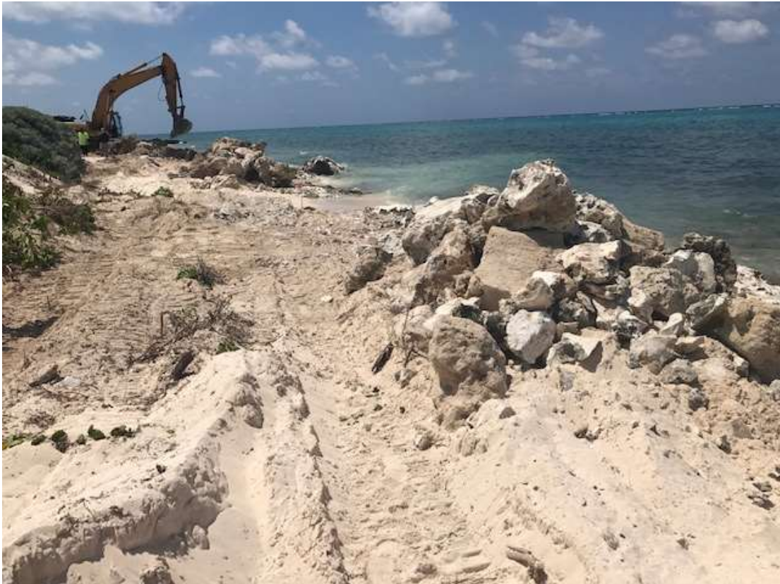
Figure 9: Stockpiling and on-land activities impacting the marine environment through turbidity and deposition of waste
